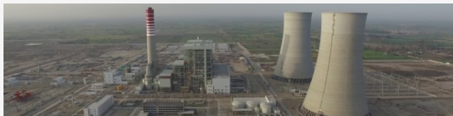
Aerial View of Sahiwal Coal-fired Power Plant
