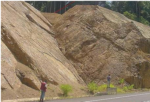
Wedge Failure
